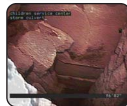
•• Service Center Storm Culvert
