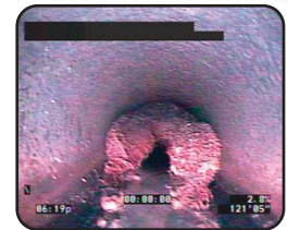
•• Severe Root Blockage
